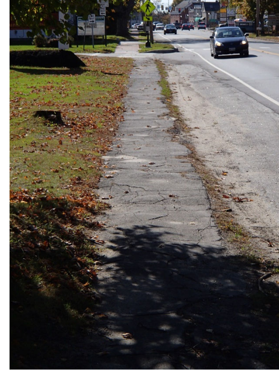
An existing sidewalk adjacent to Pennell is narrow, crumbling, and needs re-surfacing.
