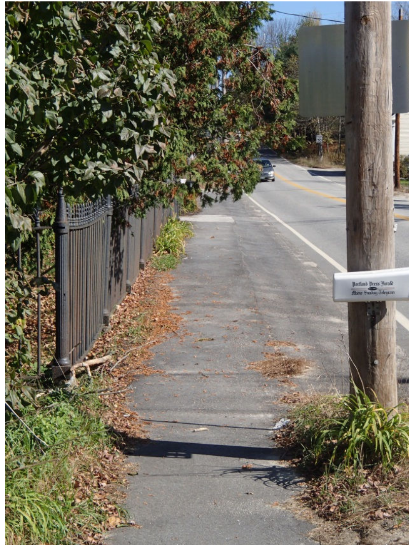
The Yarmouth Road (Route 115) sidewalk is narrow and uneven in places, and does not extend very far outside of the village center.
