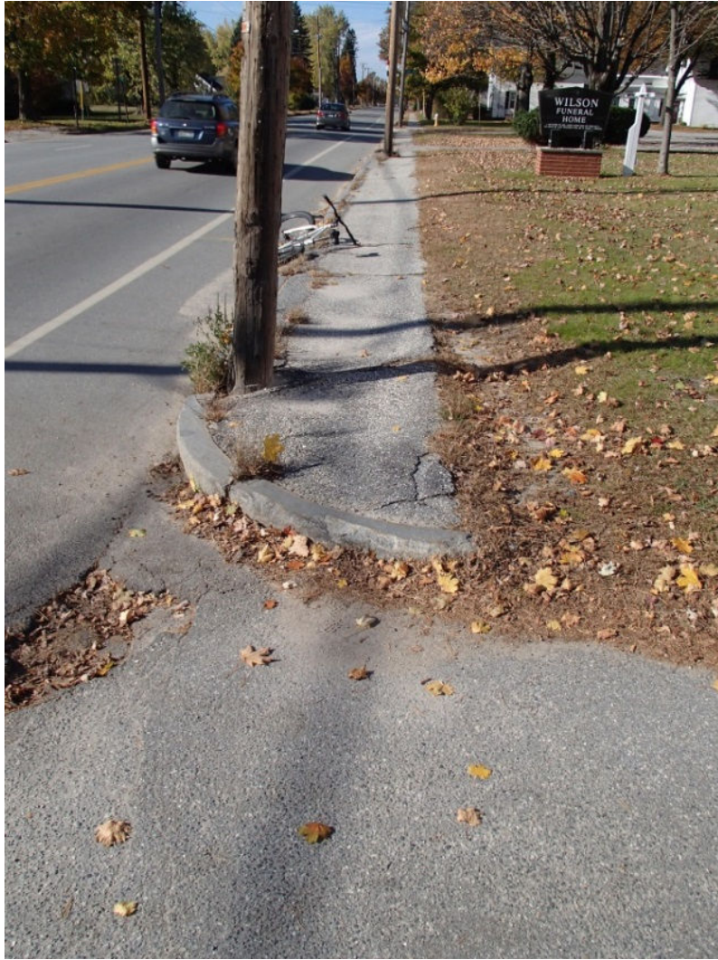
This sidewalk on Shaker Road (Route 26) is narrow, cracked, and lacks accessibility features.
