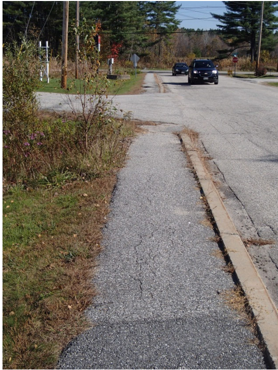
The sidewalk adjacent to the new Post Office is narrow and cracked, with no sidewalk across Rte. 100
